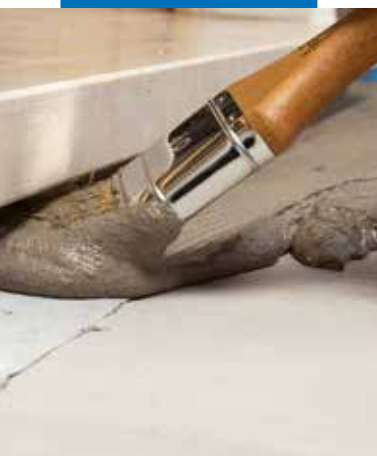
Application of Mapeband SA in difficult areas, such as under a doorstep
