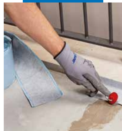
Application of Mapeband SA around edges
