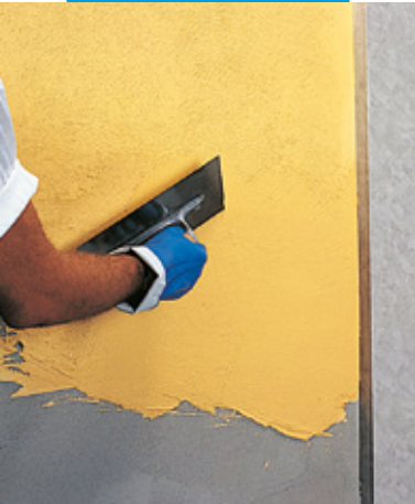
Applying Silexcolor Tonachino with a trowel
